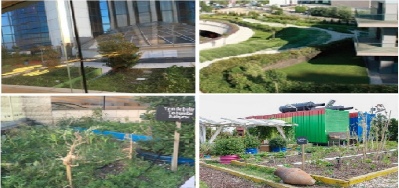
Examples of Green Roof applications (various shopping malls in Istanbul)
